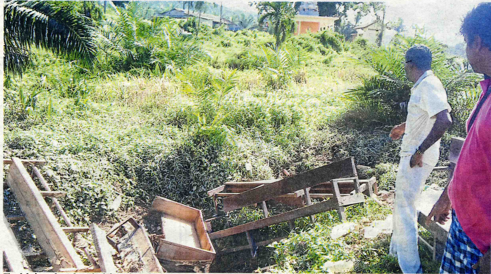
The debris and mud washed down by a downpour near St Anthony Chapel in Desa Coalfield, Sungai Buloh.
