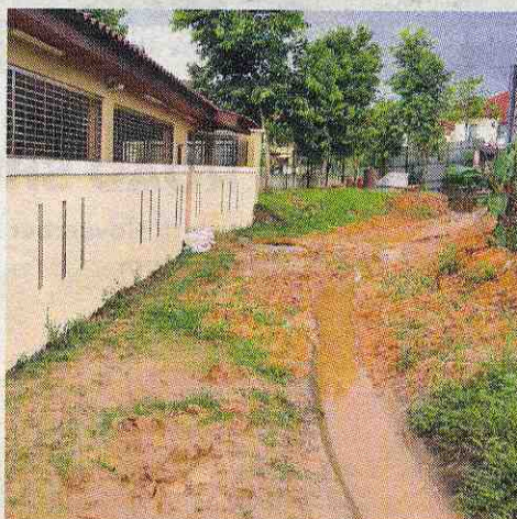
No flow: The drains behind the house are clogged by mud and stone run-off from a nearby housing development.
