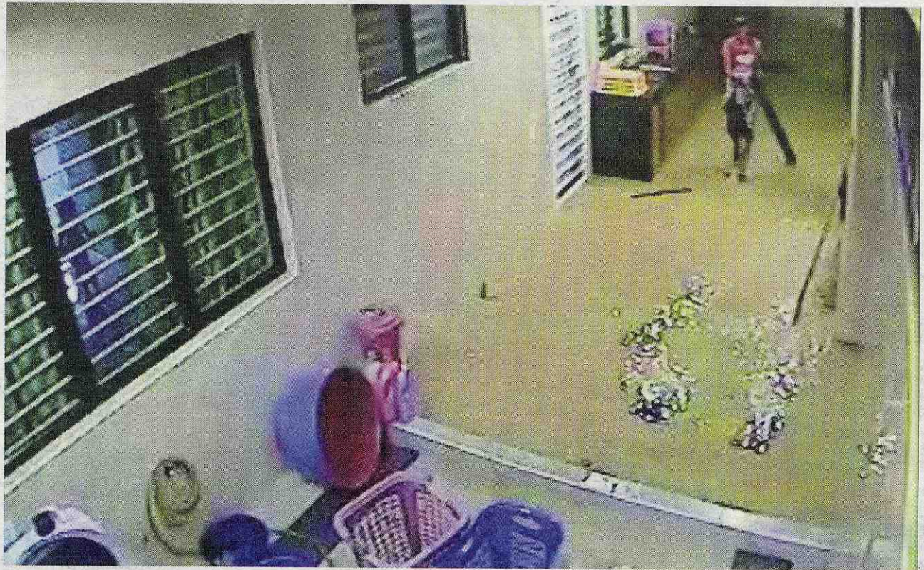
Shocking: A CCTV image of Thiagarajah's kitchen flooded after the last downpour. — Photo courtesy of resident.
