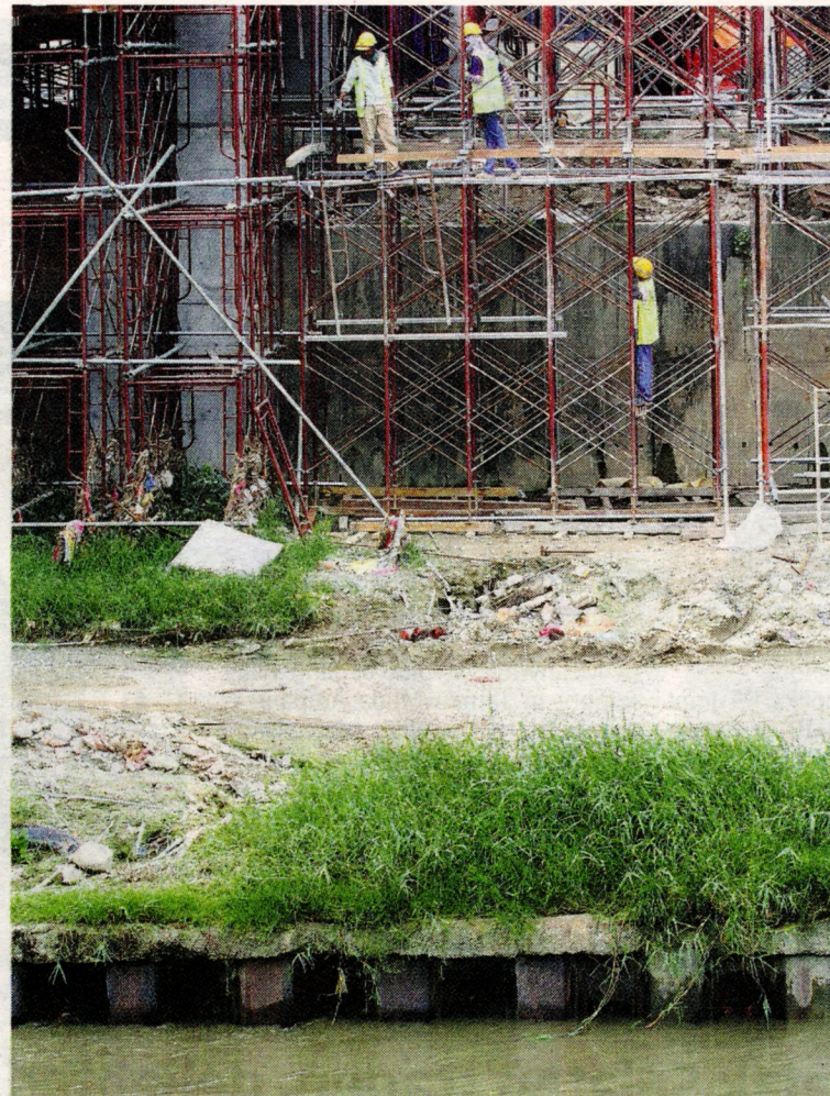
Depot in the making: Works along the riverbank is part of the Monorail Fleet Expansion Project.
