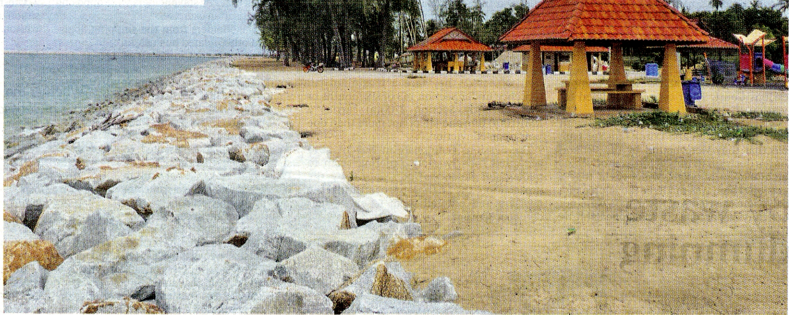
The Kampung Tok Jembal beach is safe from erosion, thanks to a granite seawall constructed by the Department of Irrigation and Drainage.
