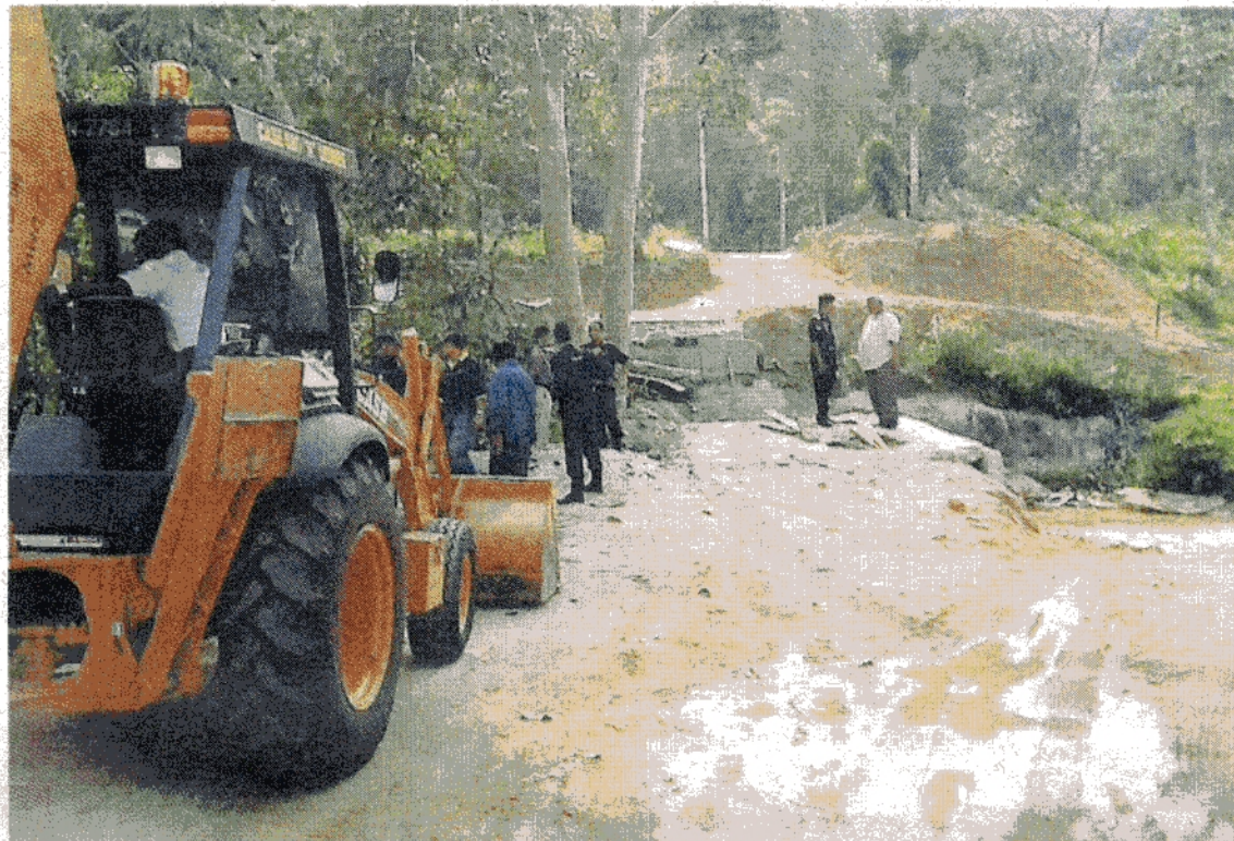
Ready for action: A backhoe on standby with authorities ready to demolish the bridge leading to the resorts.
