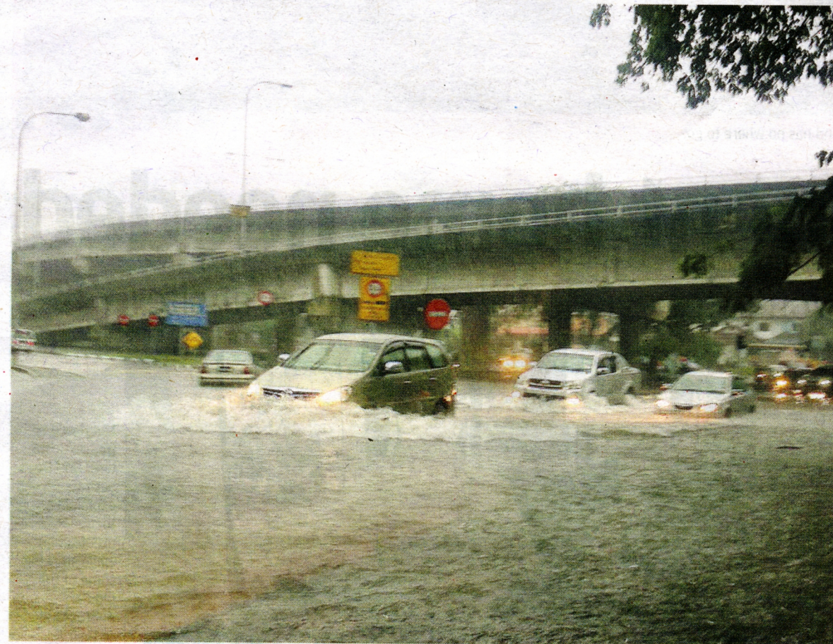
Inundated: The roundabout in Taman Midah flooded after a downpour.
