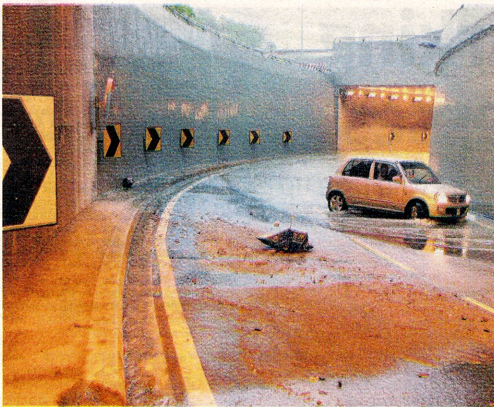
Stranded: The Cheras underpass was flooded due to the heavy rain.
