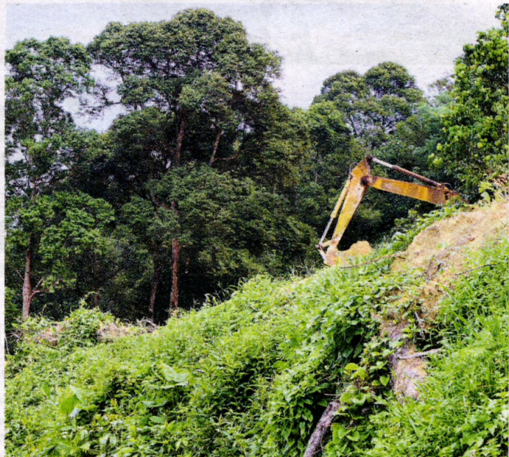
At work: An excavator digging up earth which will be transported to a washing area.
