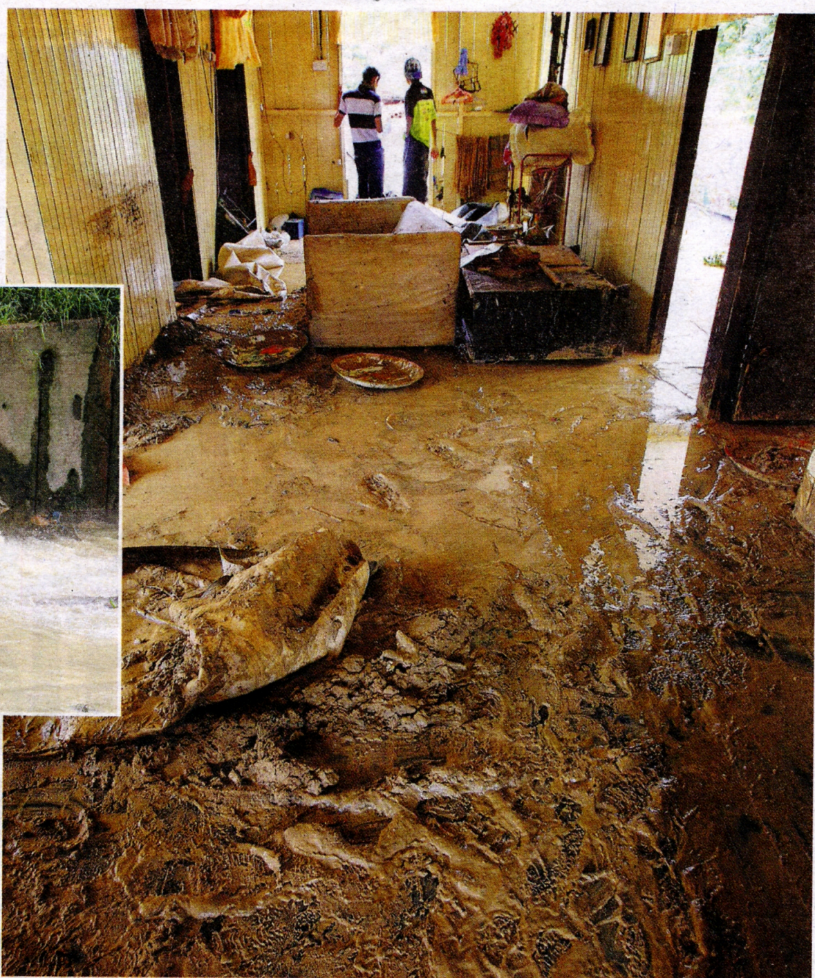
Messy aftermath: Flash floods in Kuala Lumpur early last month caked this house in Kampung Lembah Jaya Utara, Ampang, in a thick layer of silt. The frequency of floods in urban areas is increasing as drainage systems cannot cope with massive stormwater runoffs.
