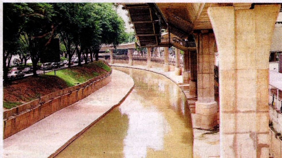
Sungai Klang looks more like a huge drain rather than a river, as its meandering banks have been straightened and covered with concrete to enable speedy water flows.
