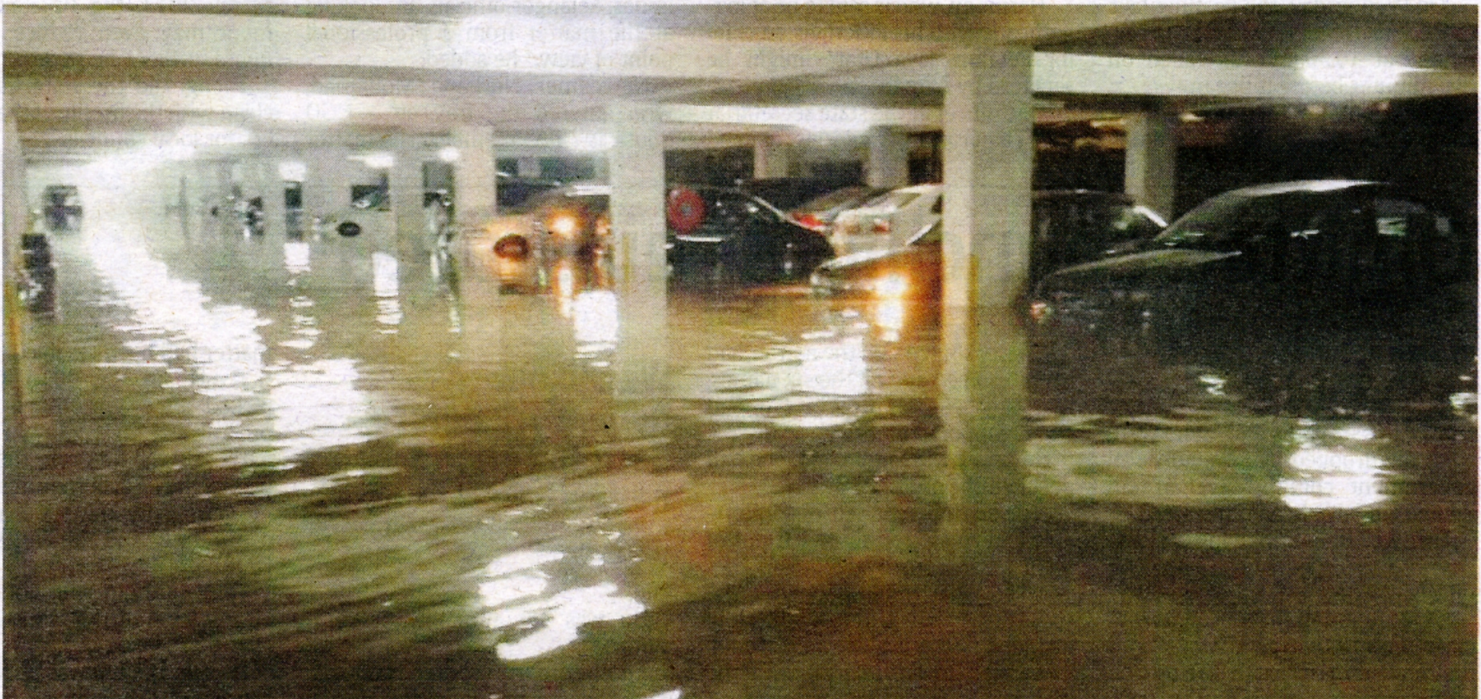
Water, water, everywhere: The car owners at USJ One Avenue Condominium were not informed about the floods.
