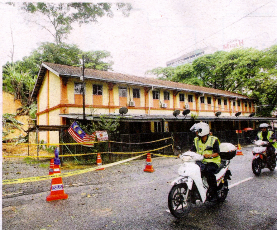
Fatal landslide: Guards patrolling the landslide area at Jalan Belfield in Kampung Attap where Raja Mohd Irfan was trapped in heavy mud before he died at the Kuala Lumpur Hospital.
