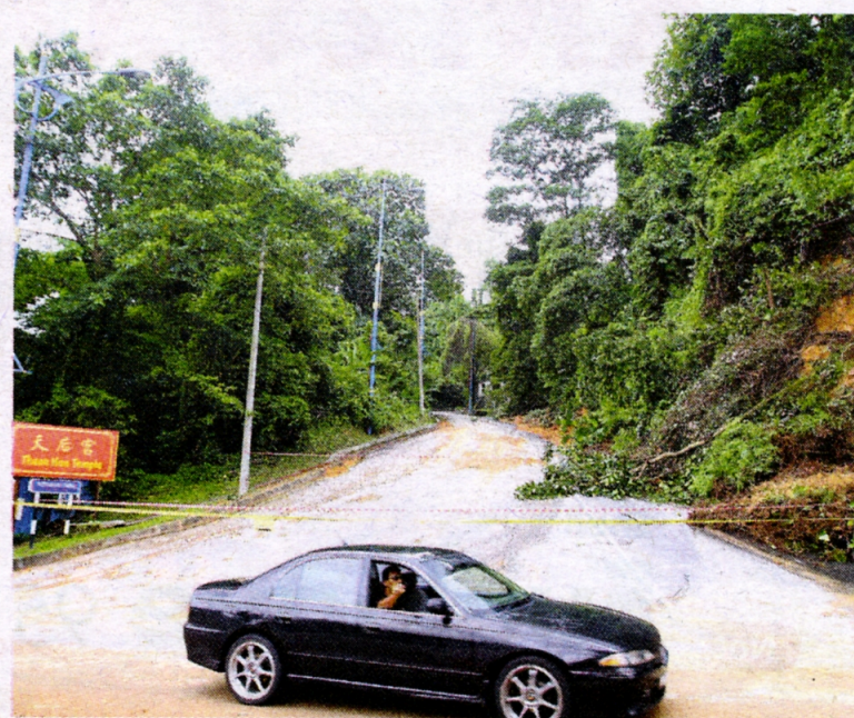
Slippery slope: The stretch of road leading to the Thean Hou temple in Kuala Lumpur was cordoned off.
