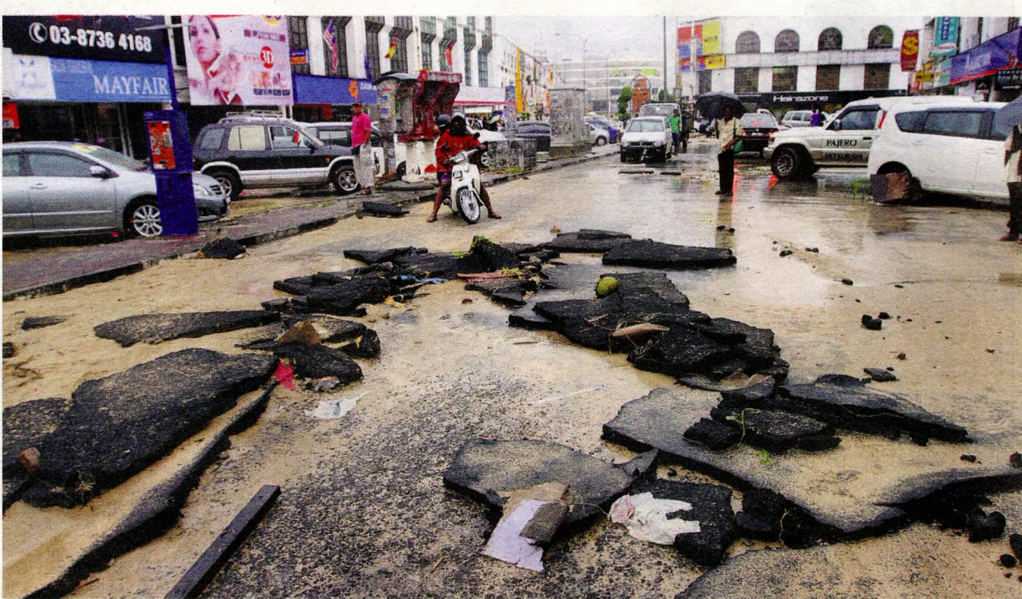
Taken by surprise: Roads were badly damaged after a flash flood hit Kajang town on Dec 2.
