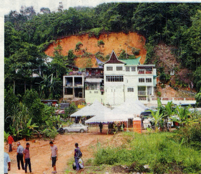
Devastating: The Hulu Langat landslide the Al-Taqwa orphanage claimed 16 lives.
