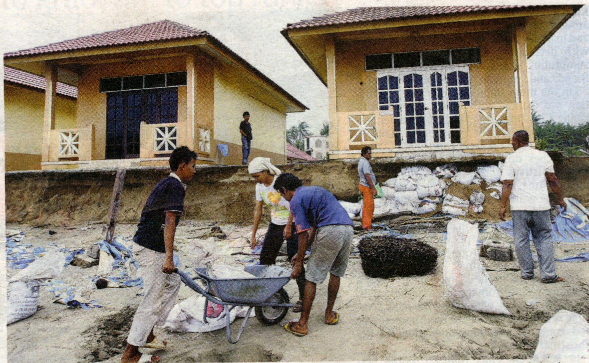
Prep work: Villagers using sand bags to shore up the edges of chalets to prevent soil erosion at Kampung Pantai Chat in Bachok yesterday. — Bernama
