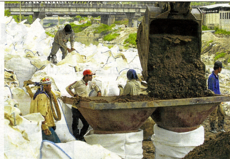
Workers carrying out dredging works along Sungai Kerayong in Kuala Lumpur. Pic by Aizuddin Saad
