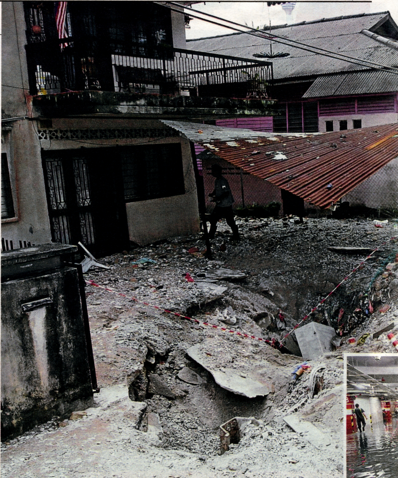
The front yard of a house in Jalan Syed Mahadi, Kampung Baru , Kuala Lumpur, collapsed after heavy rain and floods on Tuesday. (Inset) Car owners wading through floodwaters to get to their vehicles at the basement car park of Sungei Wang Plaza in Bukit Bintang, Kuala Lumpur. Pix by Zulfadhli Zulkifli
