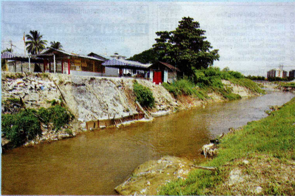
Parcel B of the Ampang Waterfront project involves this stretch where the two temples are located.
