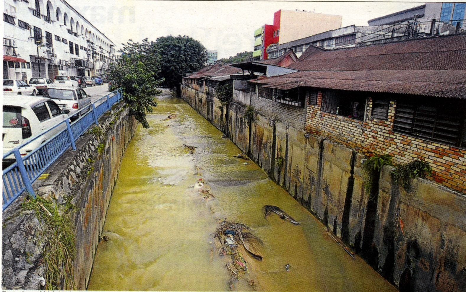
Excessive rubbish in the river near Metro Kajang shopping complex also contributed to the flooding of Kajang town on Friday. Pic by Effendy Rashid
