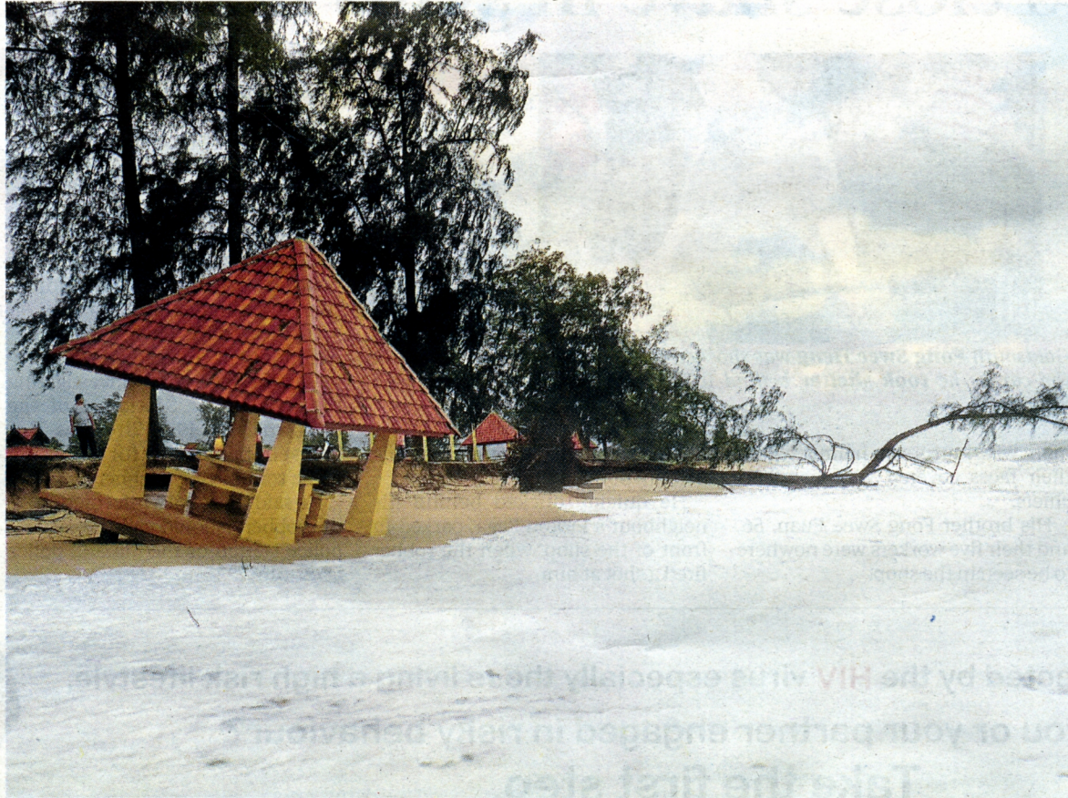
One of the four gazebos at the Tok Jembal beach in Kuala Terengganu that was destroyed by strong waves yesterday. Pic by Satiman Jamin
