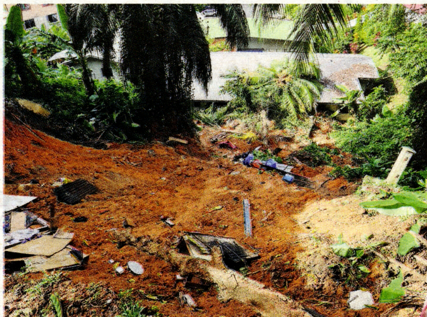
On shaky ground: A wooden house on the verge of collapsing after a heavy downpour caused a landslide in Kota Kinabalu last night. - Bernama
