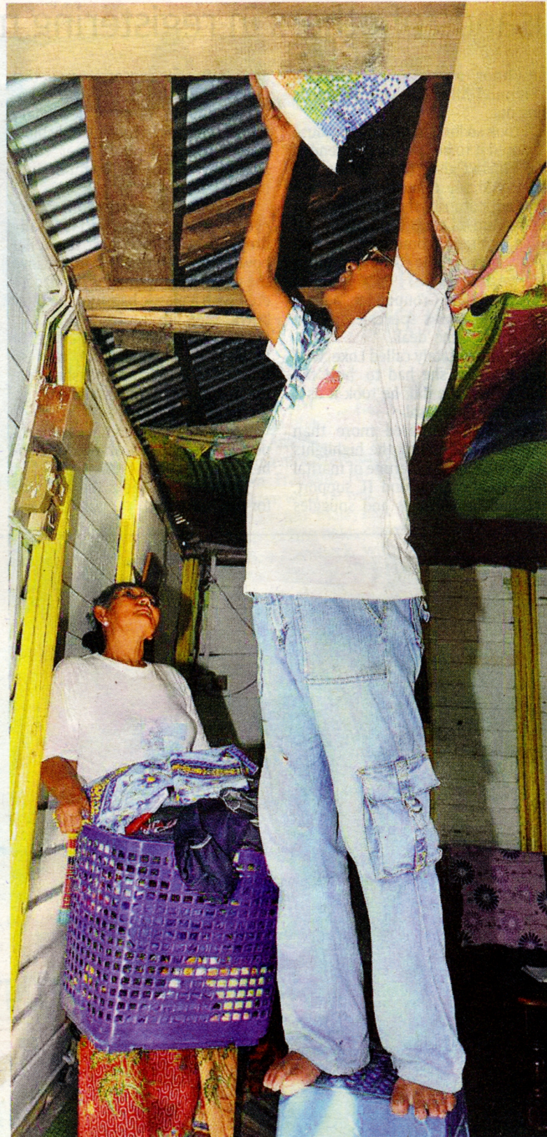
Not taking chances: Atan and his wife Aminah Mat Ali, 58, storing some of their valuables inside the newly-installed wooden shelves at his house in Taman Mawai.
