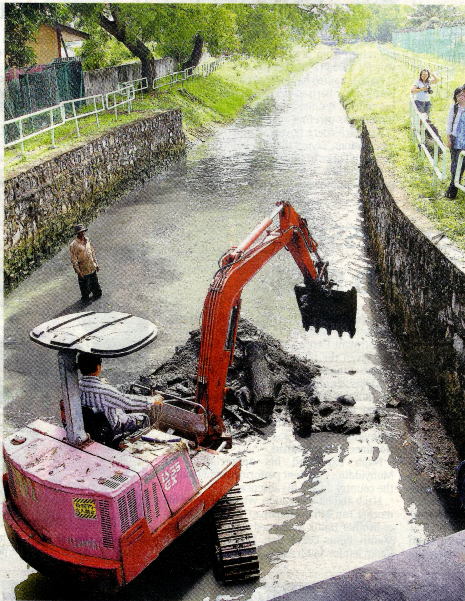
Digging in: Dredging work being carried out in Sungai Gelugor, Penang. The second phase to deepen the river started on Tuesday as part of efforts to mitigate flood problems.
