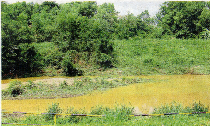
Poor maintenance: The retention pond which overflowed last Friday after a two-hour downpour.
