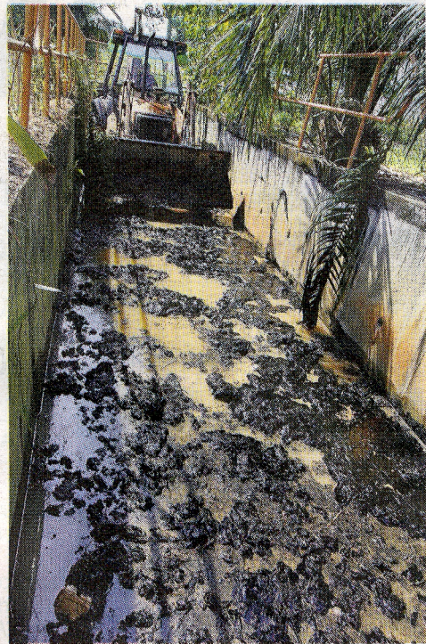
Clean-up: An excavator clearing the oil sludge from a monsoon drain in Port Dickson yesterday.
