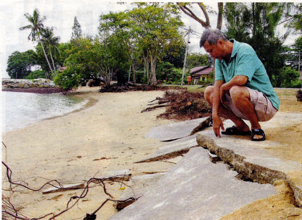
Encroaching sea: Koo examining the damage to the court along Tanjung Kling on Friday as a result of recent rapid beach erosion.
