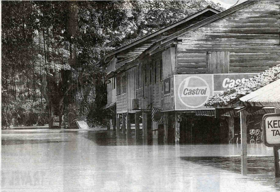
Inundated: High-level floodwater affecting the small town of Panchor in Johor recently. Residents and traders in the town have been given time to pay assessment taxes and renew business licences this year.
