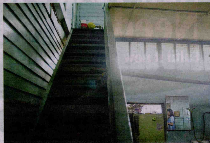
Stairway to safety: A staircase leading up to the roof (below) is also a common addition to the houses in the village.
