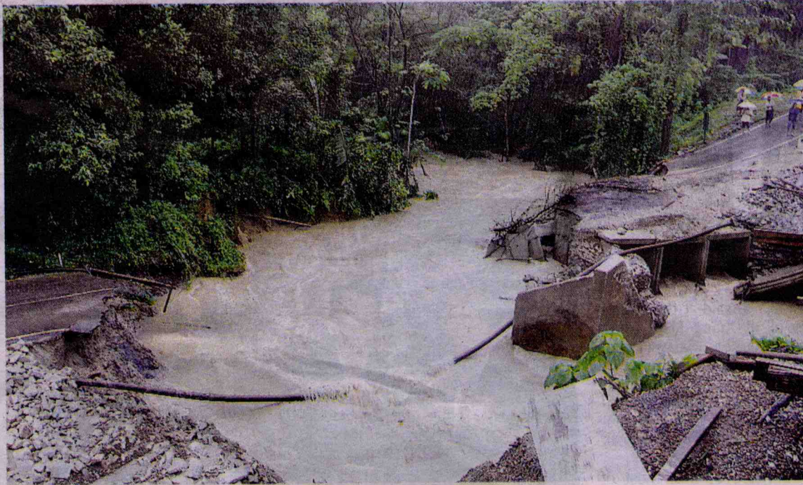
Damaged again: The bridge connecting Kampung Dura and Jenagor in Terengganu was washed away due to strong currents for a second time. The previous bridge was washed away last year. — Bernama
