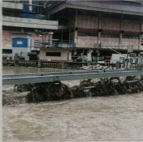
A poor drainage system is a major cause of flash floods in the Klang Valley. FILE PIC
