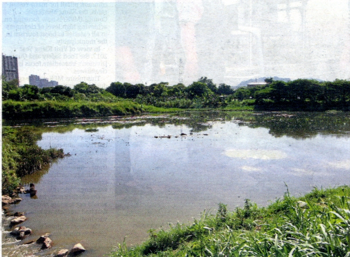
The water retention pond at Taman Sri Serdang that will be upgraded.
