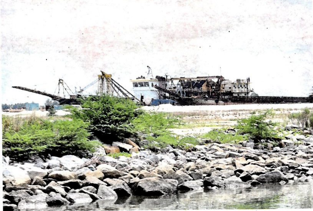
Reclamation work carried out in Tanjung Kling recently.
