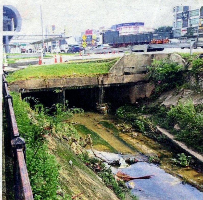
Sazally says unlike a single-cell box culvert system, the triple-cell box culvert system is more prone to being clogged with mud, obstructing water flow.
