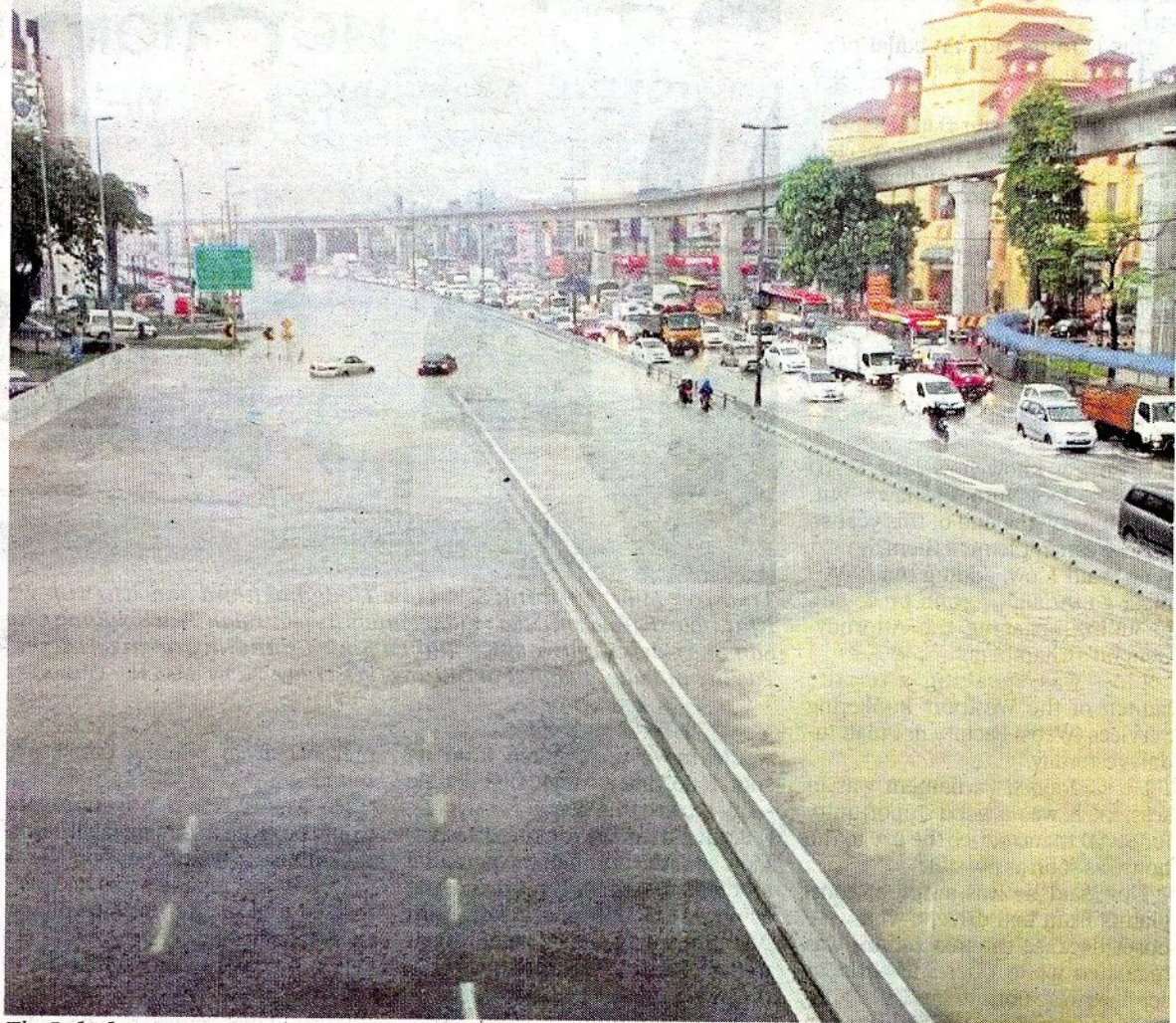
The Lebuhraya Damansara-Puchong stretch near IOI Mall was inundated yesterday after heavy rain. Pic courtesy of reader
