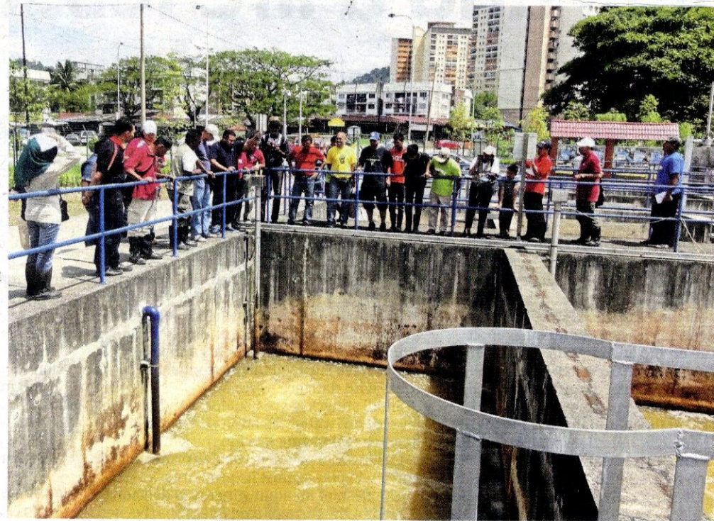
The community leaders being briefed on the water treatment process at the Sungai Sering River Water Treatment Plant in Ukay Perdana, Ampang.
