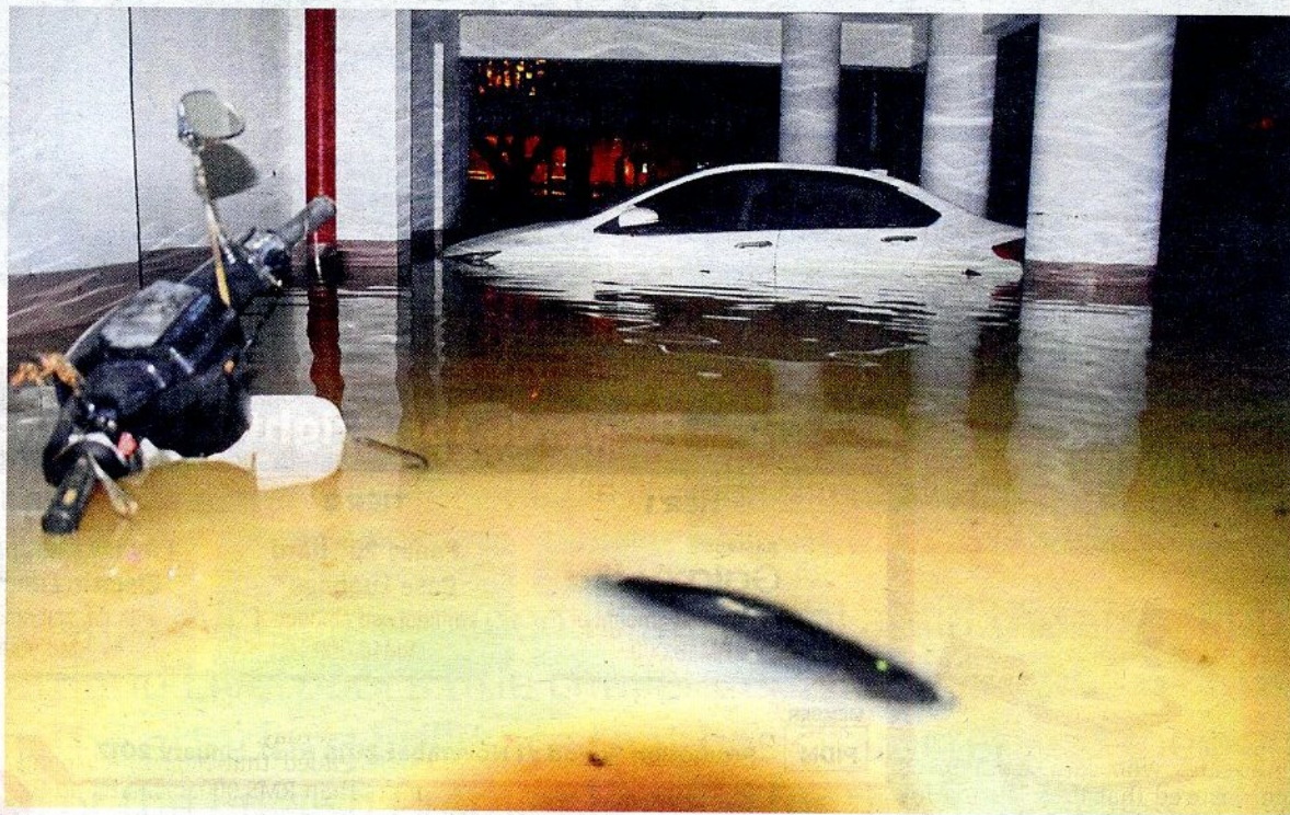
Drowned: A motorcycle and a car found submerged by the flood in an underground carpark of an apartment in Sungai Dua.
