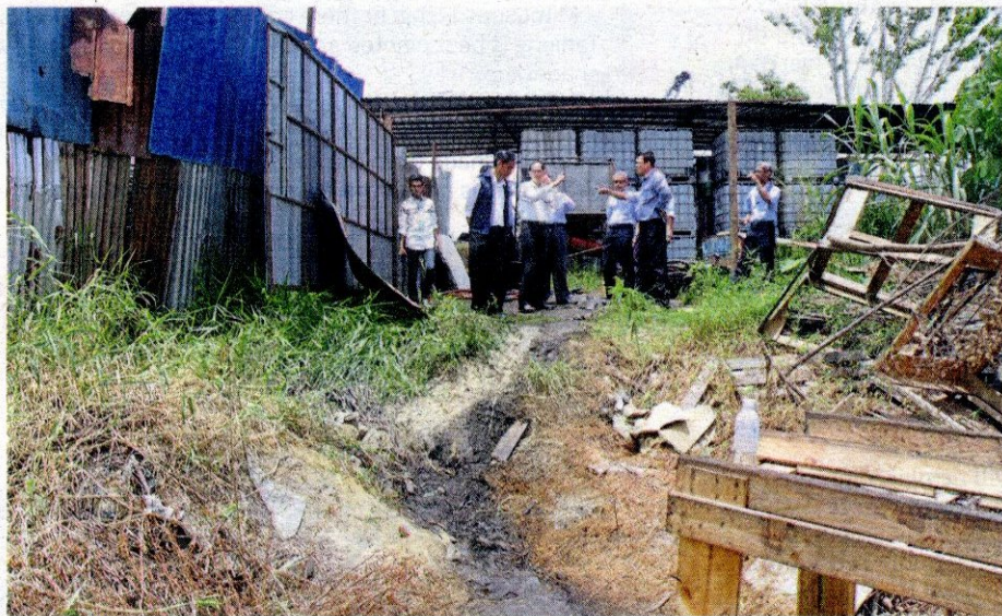
Kajang Municipal Council officers visiting the site of the factory in Jalan Sungai Lalang, where contamination from the factory had leaked into Sungai Semenyih. — filepic
